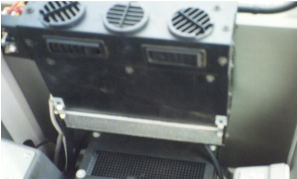
Evaporator assembly mounted in place.
